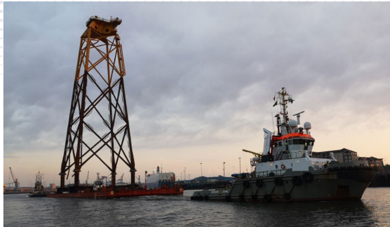
WTG jacket foundation (50m water depth)
