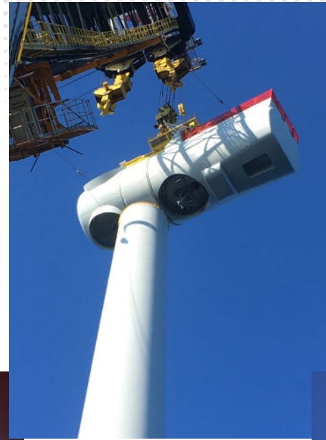
Nacelle lowered onto tower
