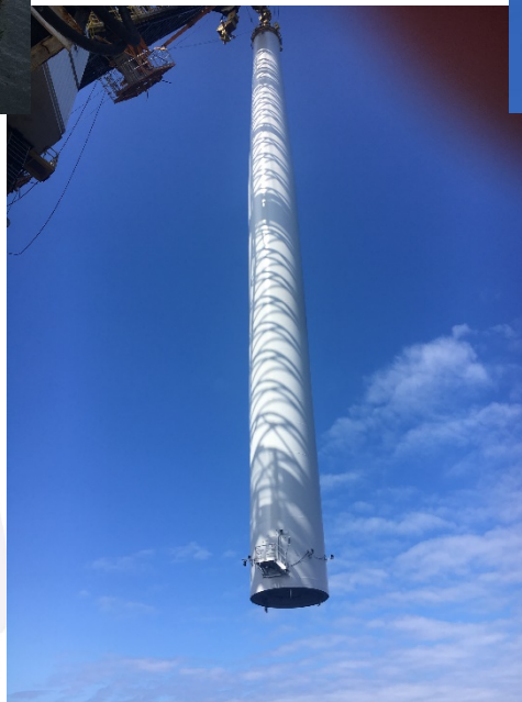
WTG tower lifted onto TP
