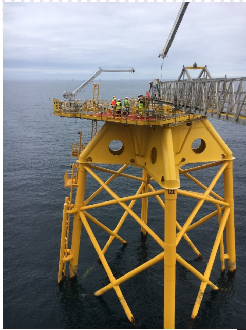
Jacket (including transition piece)
