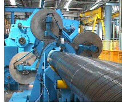
Application of Flextape™
