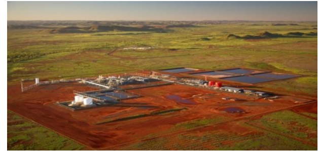
Devil Creek domestic gas plant, Cape Preston, WA.
