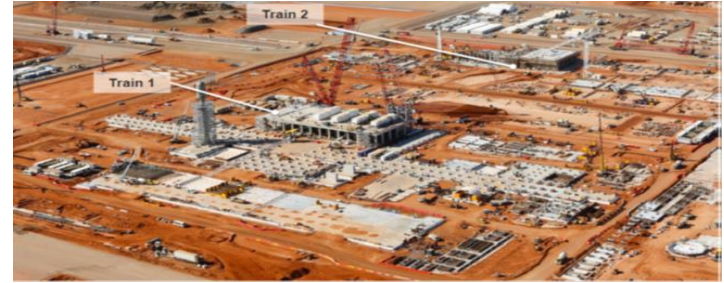
Wheatstone LNG plant construction, Onslow, WA. Image: Chevron
