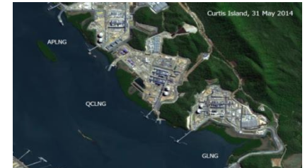
3 projects & 6 trains LNG, Gladstone, Qld. Image: Santos
