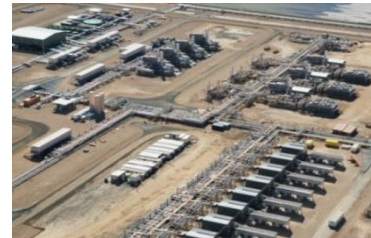
Well head production, gathering, stabilisation. Image: Santos
