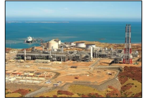
Pluto LNG plant, Burrup Peninsula, Karratha, WA Image: Woodside
